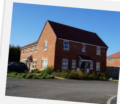
Affordable New Build Housing at East Shaftesbury
